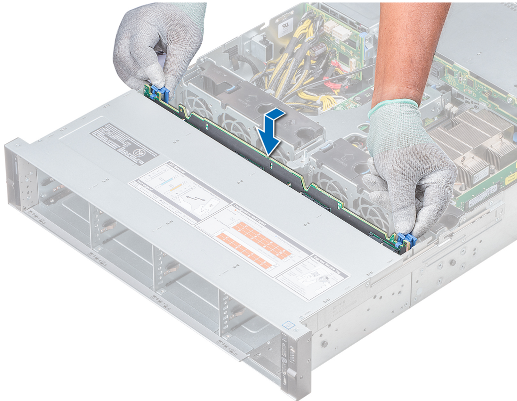
Figure 102. Installing the backplane
