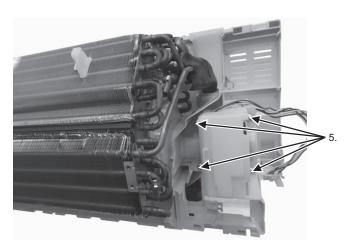
Remove 4 screws from fan motor cover.
